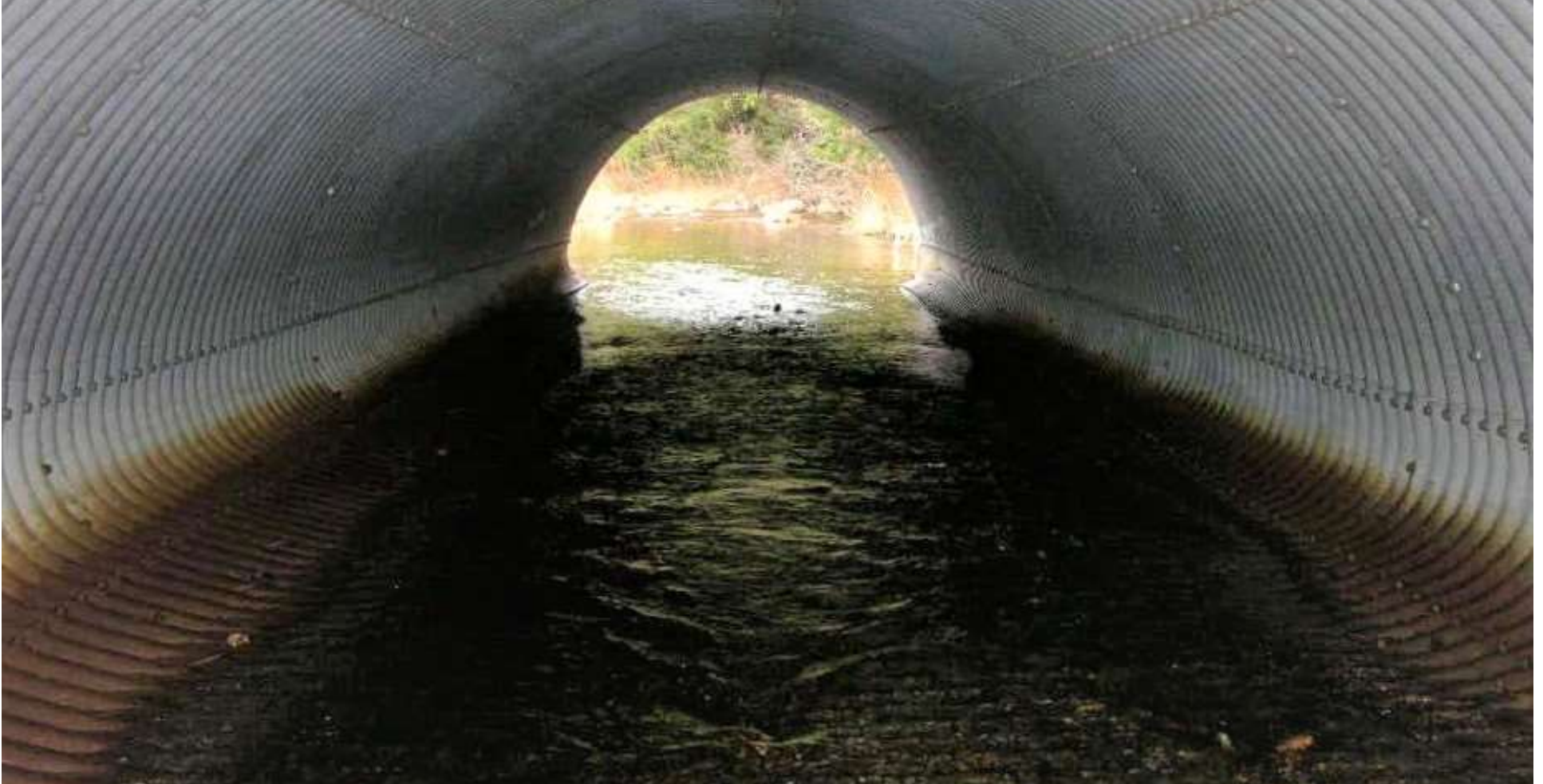
Typical Corrosion Deterioration
